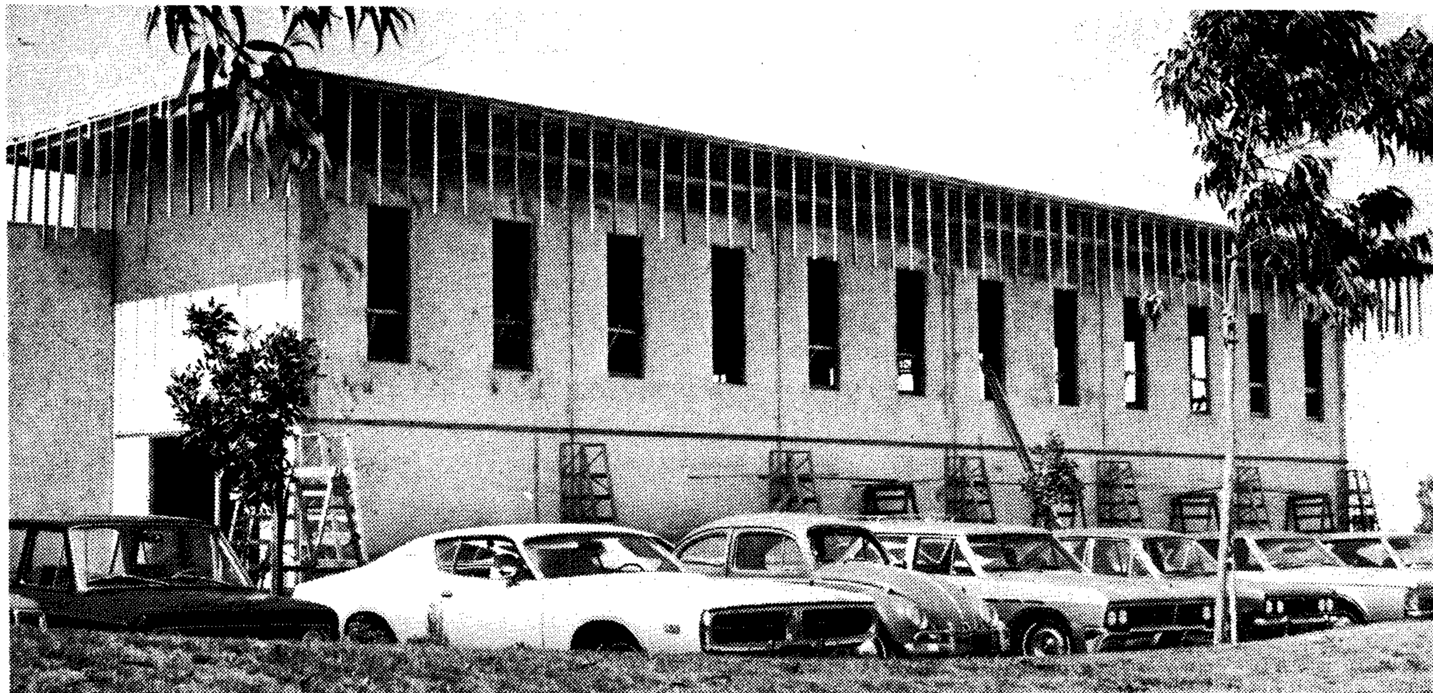
MICRODATA'S 48,000 sq. ft. addition moves along on schedule. When completed in early 1975, it will double the company's current plant size.
